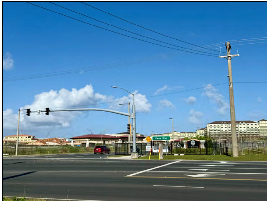
Construction continues on the new Marine Corps Base Camp Blaz.
